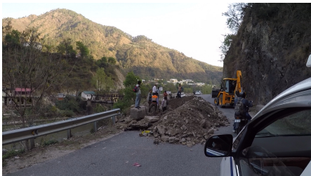
Figure 1: Construction on the road in Kamand on March 27, 2018.
