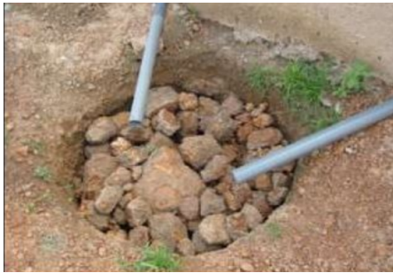
Figure 6: Soak pit in Katindi
