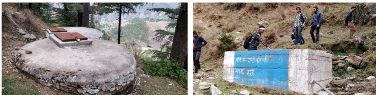
Figure 5: Water Tanker at Arnehar village
