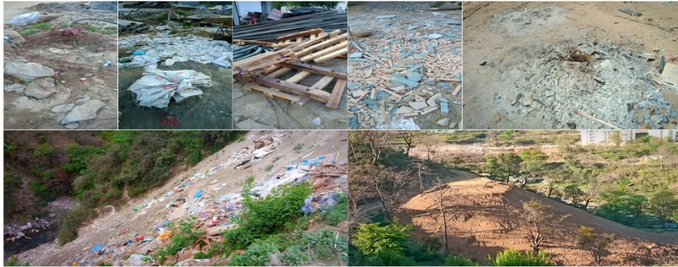
Figure 5: Construction waste management in campus
